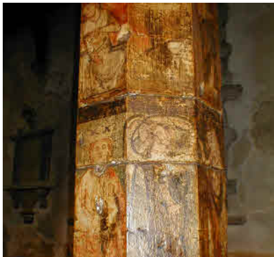
The painted column 1306
